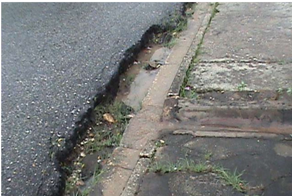
Below: The edge of the road where at least two vehicles became stranded
